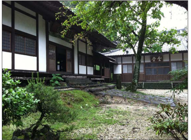
Shogoji Hatto (Dharma Hall, left bldg.) and Sodo (or Undo, Monks' Hall, right bldg.) Photo by Erin Davis.
